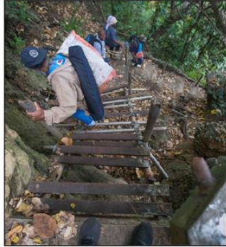
Above Left: Make-shift steps created by villagers on footpath with sticks and rope between Matangi and Ipau; Above Right - descending damaged steps without railing near Marae village in Matangi (PC - Niki Kuautonga)
